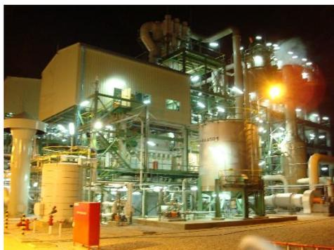
The PVC slurry from the VCM Removal section is fed into the centrifuge continuously in order to separate wet PVC cakes from water. The wet PVC cakes discharged from the centrifuge are dropped into a fluidized bed dryer, where moisture is removed from the PVC powder. The dried PVC powder passes through product sieves to eliminate any oversized particles, and is conveyed pneumatically to the product silos. The PVC product thus obtained maintains uniform quality.
